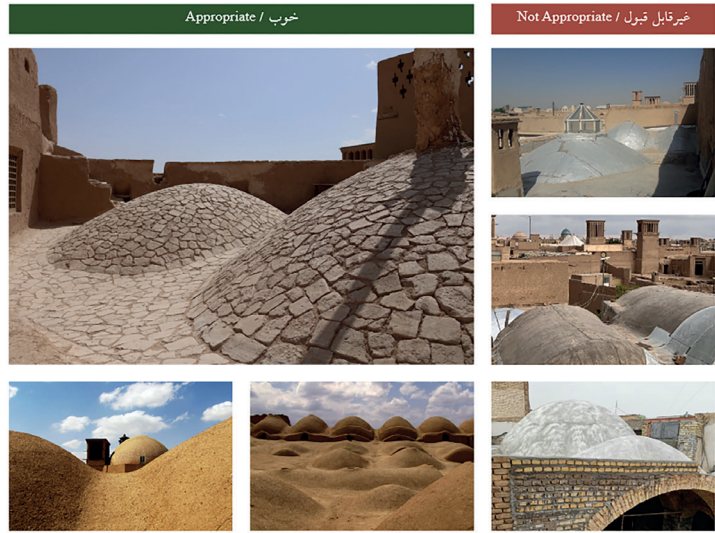
In Yazd architecture, clay property to transfer water was applied in roofs. When the sloping was properly designed on flat and curved roofs, a mixture of clay and straw was adequate without the need for brick flooring. Sometimes flat surfaces on the roof were covered with brick flooring to facilitate the use of roof space. For curved surfaces of the roof, using broken bricks from other construction operations was common.
